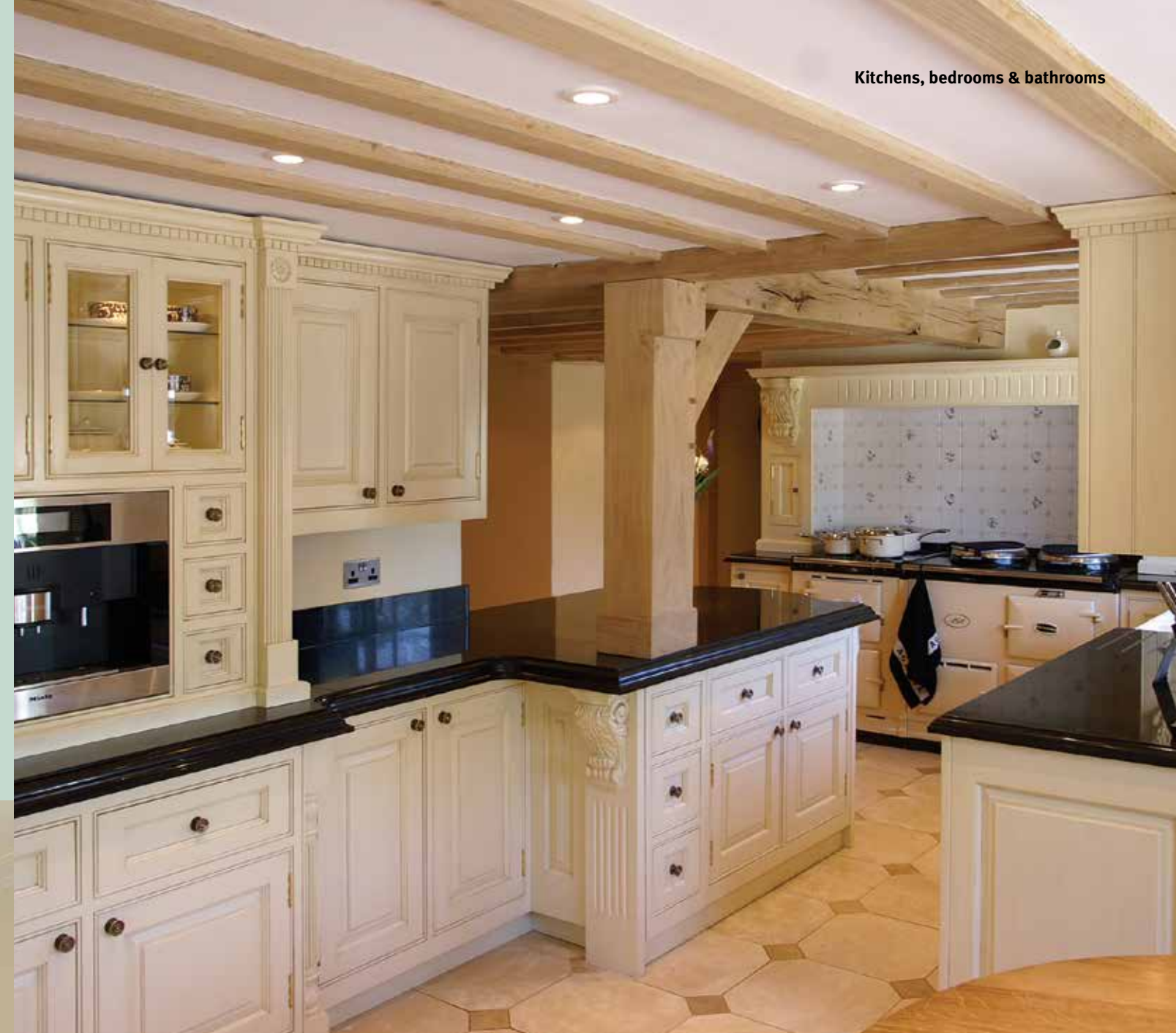
The kitchen above was part of an extension to a 16th century oak-framed Wealden Hall house. The false ceiling beams are made from Orlestone air-dried oak, and the structural steel post was enclosed in a hollowed-out oak beam
