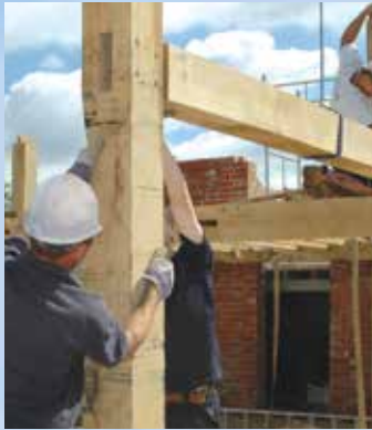
The oak frame was built around the brick kiln.
