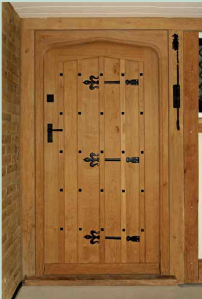
EX01: Traditional arch-topped solid oak door and frame with fillets and traditional ironmongery and false hinges.
