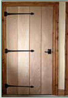
IN01: Ledge and brace oak door. To achieve a higher fire rating 32mm thick ledge and braces were used.
