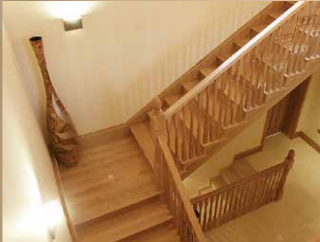
A traditional hand-carved oak staircase, stained and waxed for an antique finish.
