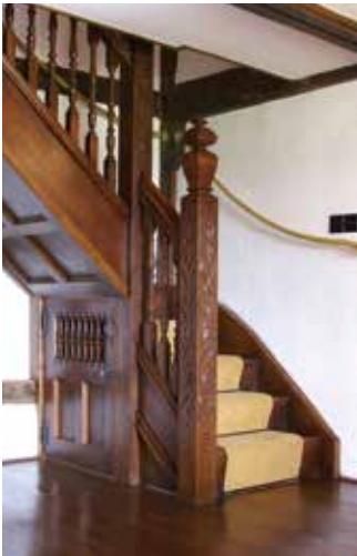
A traditional hand-carved oak staircase, stained and waxed for an antique finish.
